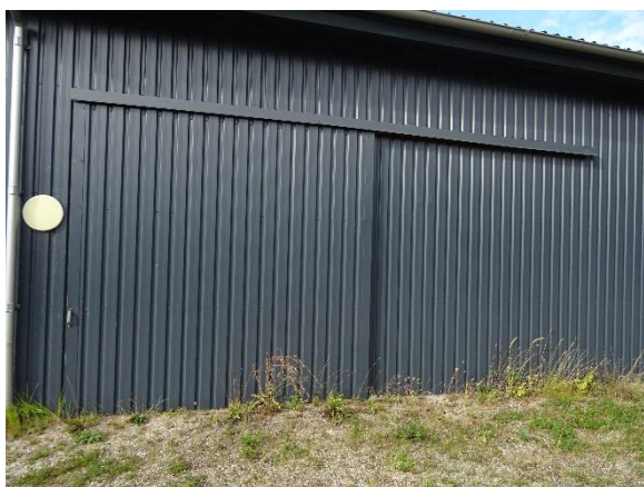
Skydeport i facade
