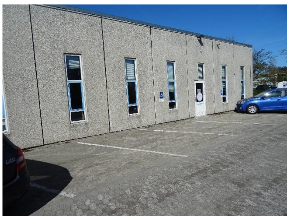
Beton sandwich facade
