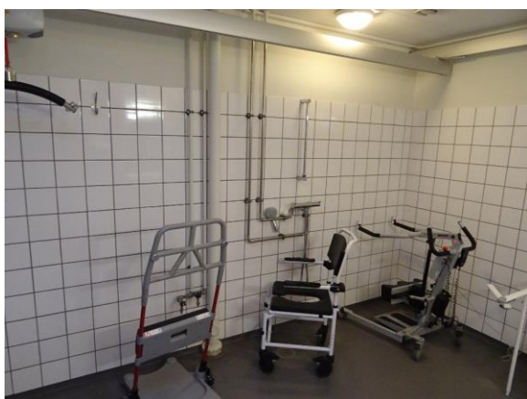
Rustfri installation i renoveret toilet/bad
