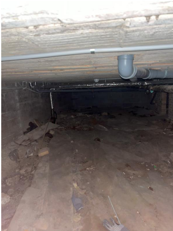
Randfundament i beton
