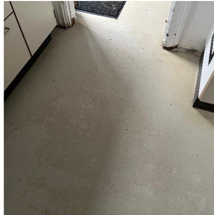
Epoxygulv, malet beton
